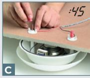
Two (2) standard wire nuts connect the speaker wires to the mounting studs, making the electrical connection. That's all it takes!
