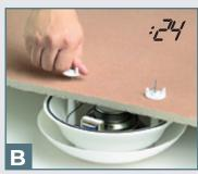
Two (2) wide-based wing nuts secure the speaker assembly to the ceiling tile.
